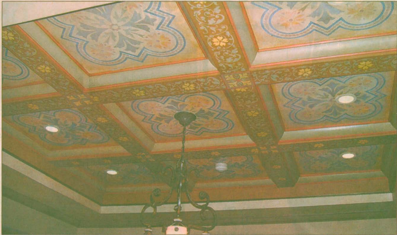
THIS COFFERED CEILING , painted by Bruno-Sears, is the artist's favorite type of "fifth wall." Stencils and paint can be used to achieve the look.
